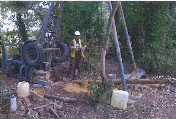
D-9 Drilling Borehole B5
