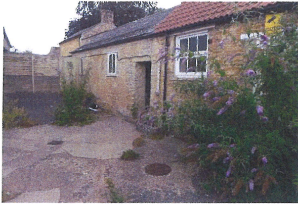
D-13 Coln House West: well located to left of doorway
