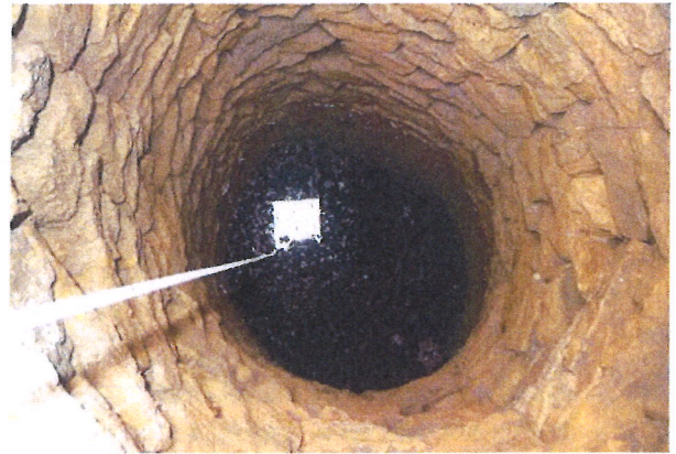
D-14 Well interior at Coln House West
